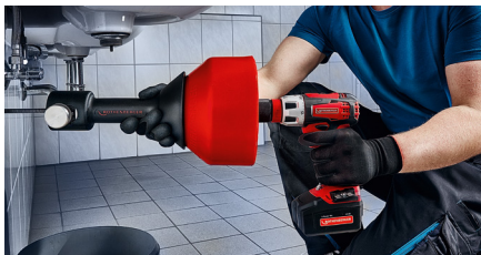
Cleaning a connection pipe of a washing basin
